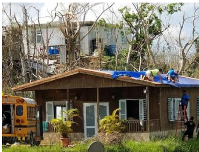
G. Lopez and his crew repairing a roof in Puerto-Rico.
